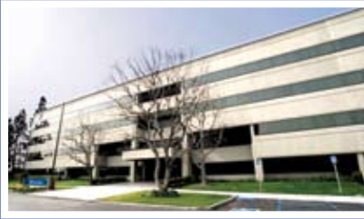
4000 METROPOLITAN Orange, CA 183,000-square-foot, 4-story office building
