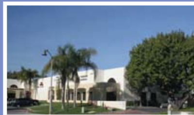
CALLE PERFECTO San Juan Capistrano, CA 45,000-square-foot industrial building
